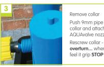
Remove collar Push 9mm pipe through collar and attach to AQUAvalve nozzle Rescrew collar - DON'T overturn... when you
